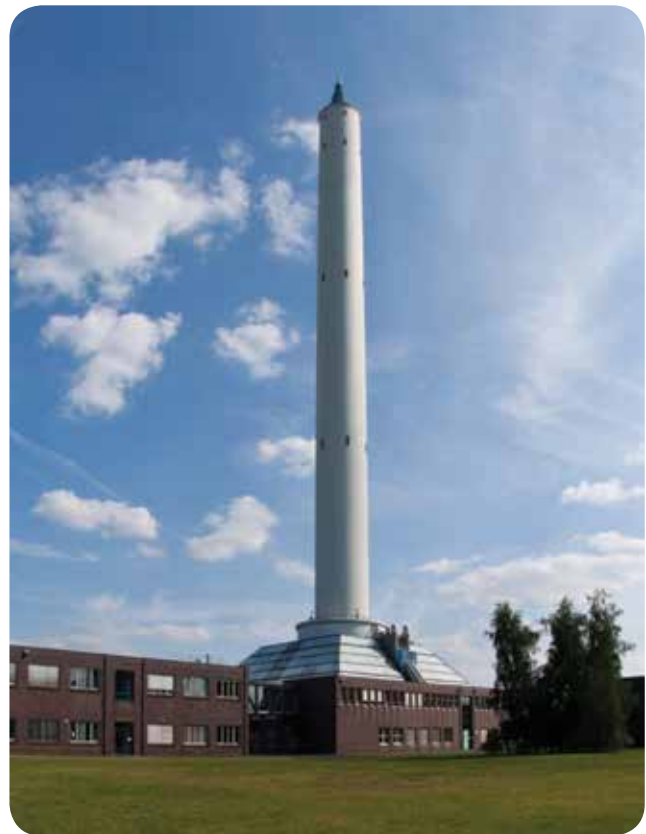
'Fallturm Bremen' is a drop tower at the Center of Applied Space Technology and Microgravity (ZARM) of the University of Bremen, Germany. It has a 123-metre-high drop tube (actual drop distance is 110 m), in which for 4.74 seconds weightlessness can be produced.
